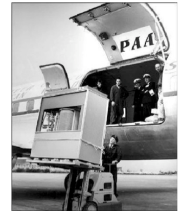
1956 IBM RAMDAC computer included the IBM Model 350 disk storage system (5M)
